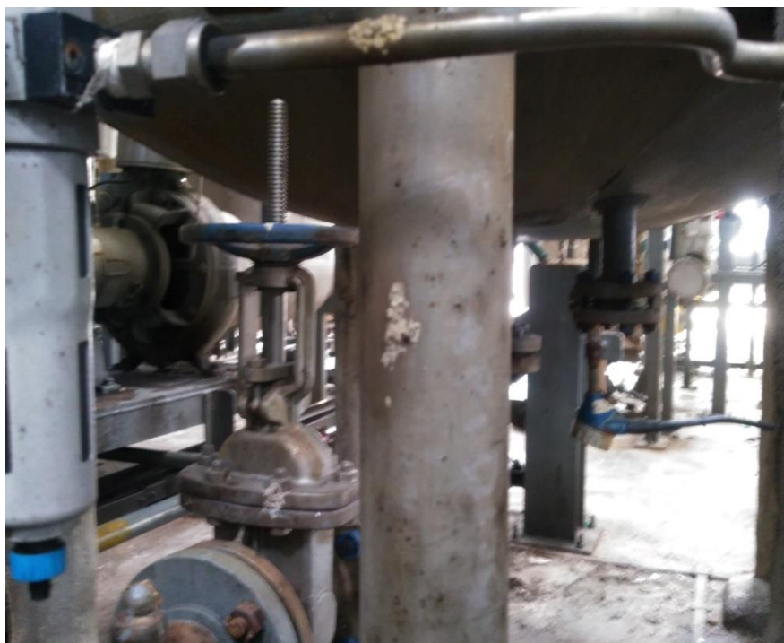
Photo 4: Column support and earthing was noted in satisfactory condition
