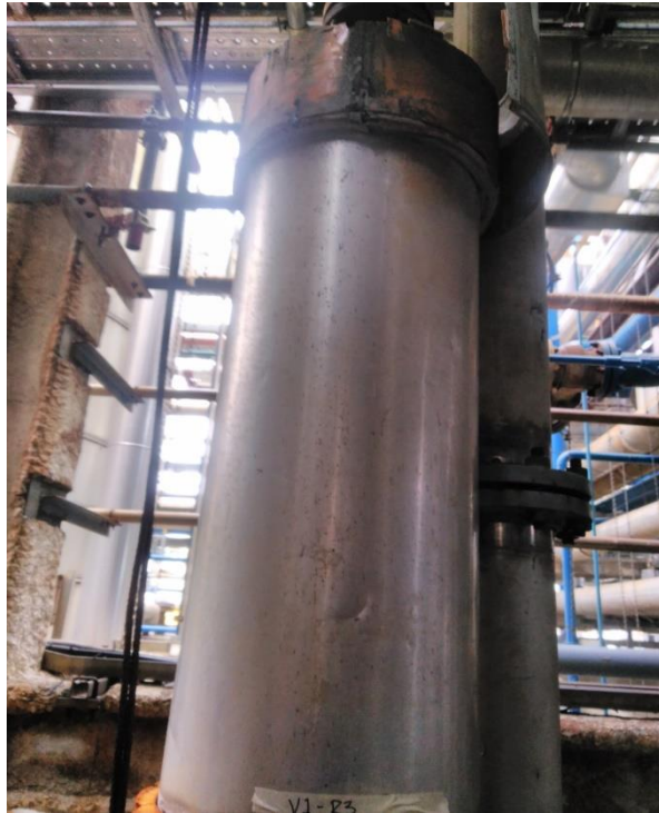
Photo 11: Top dish head pipe insulation was damaged.
