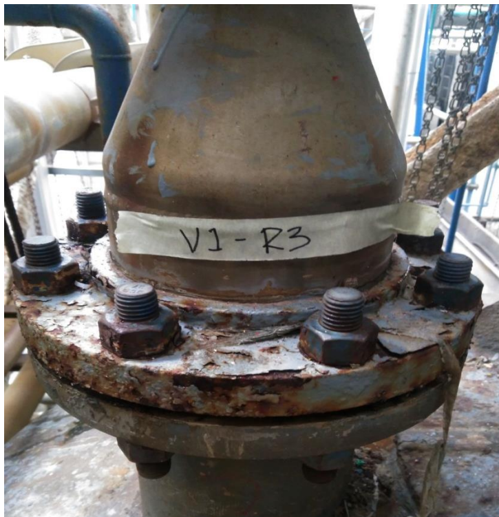
Photo 6: Top dish head nozzle was observed with minor rust.
