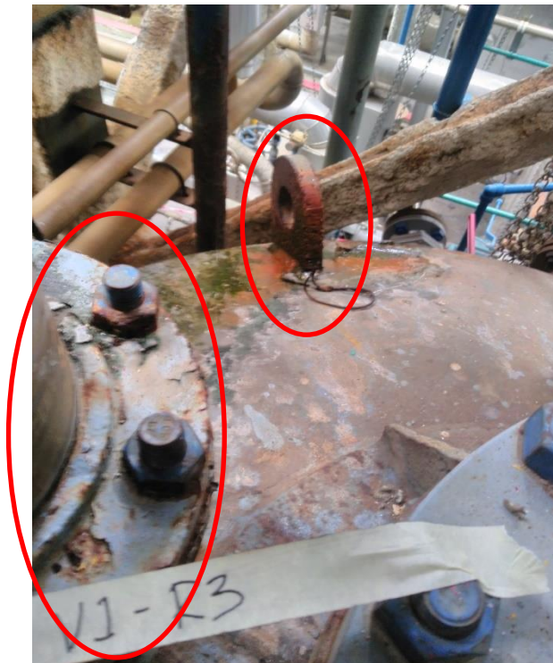
Photo 10: Top view of nozzle head. Flange was observed paint failure and lifting lug & nearby top dish head was observed with minor corrosion and algae.
