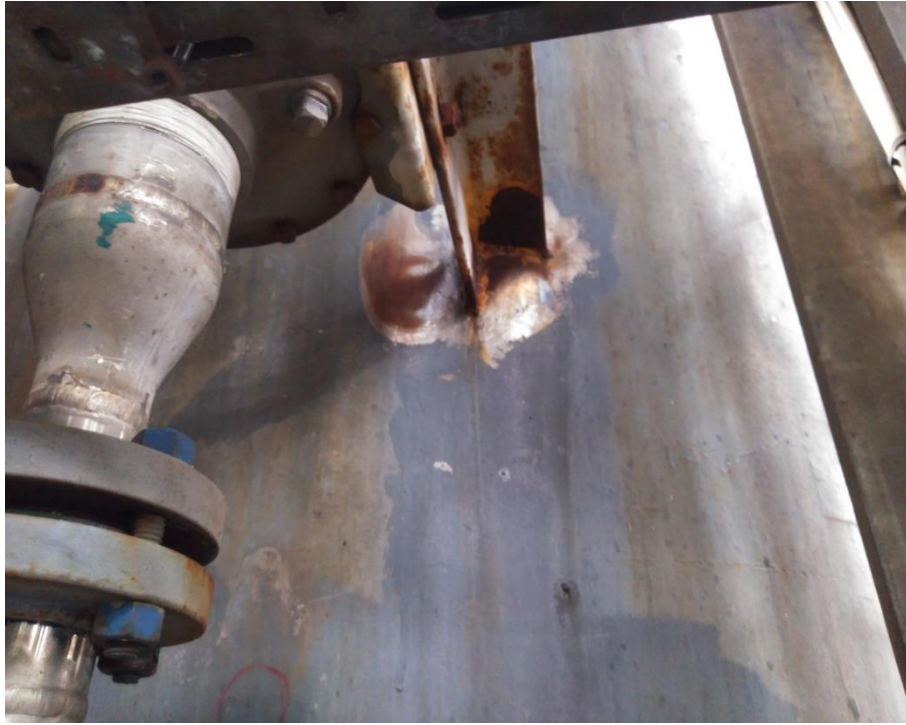
Photo 5: Pipe supports were directly welded to the shell and in satisfactory condition
