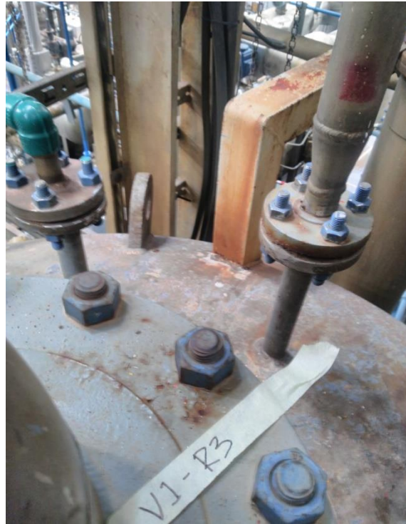
Photo 9: Shell nozzle were observed in satisfactory condition
