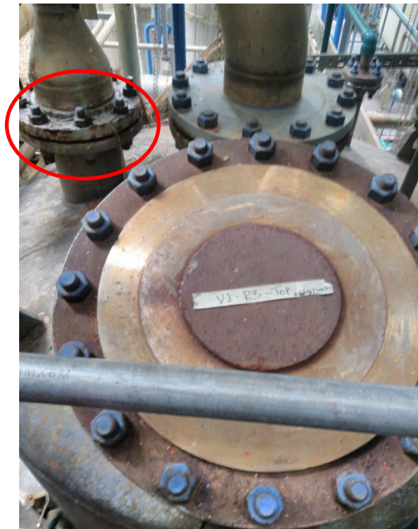
Photo 8: Top view of nozzle head. Flange was observed paint failure and lifting lug & nearby top dish head was observed with minor corrosion and algae.
